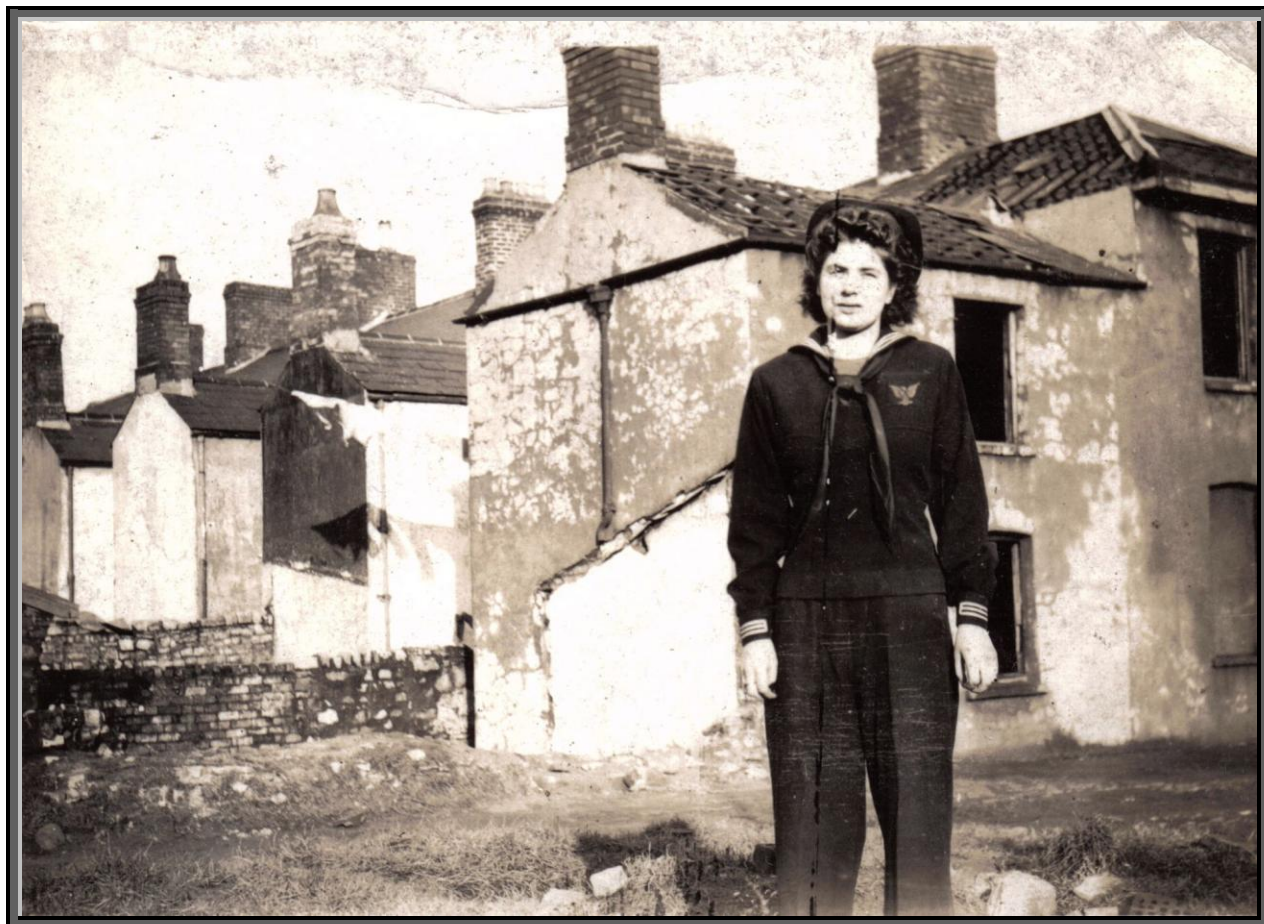
1944: Bomb damage just down the street
